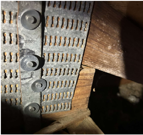
Roof to wall attachment - Clips
