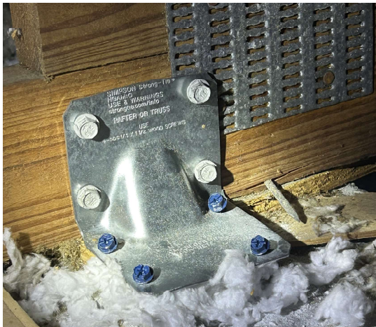
Roof to wall attachment - Clips
