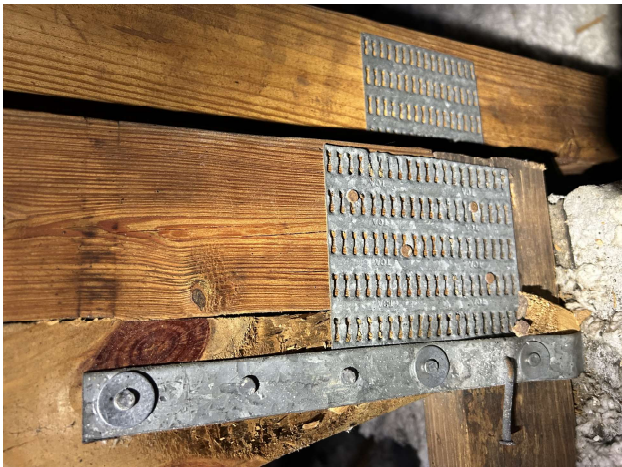
Roof to wall attachment - Clips
