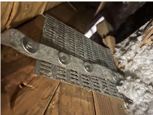
Roof to wall attachment - Clips
